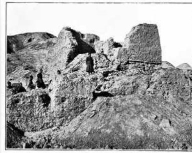
305. RUINS, M.B. I, AT MURTEK IN COURSE OF CLEARING.
